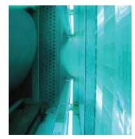
High-output UVC emitters mounted downstream from the coil destroy mold, bacteria, viruses and VOCs preventing them from re-entering the air.
